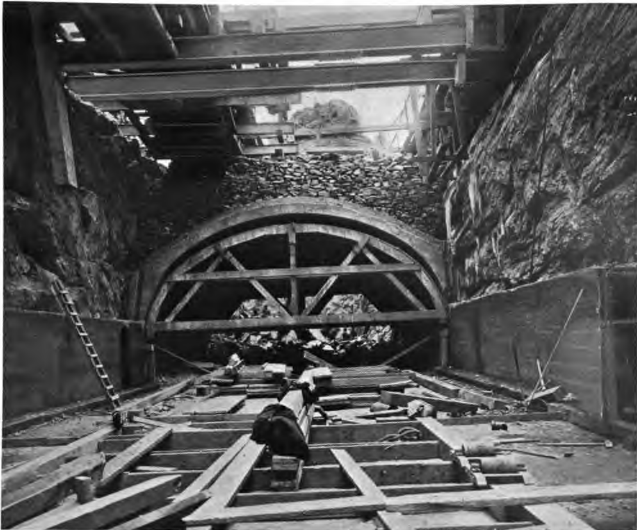
THREE-TRACK CONCRETE ARCH — 117TH STREET AND BROADWAY
